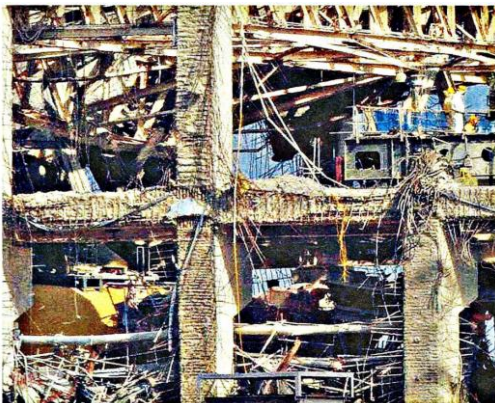
Fukushima Daiichi Reactor #4 after hydrogen explosion
