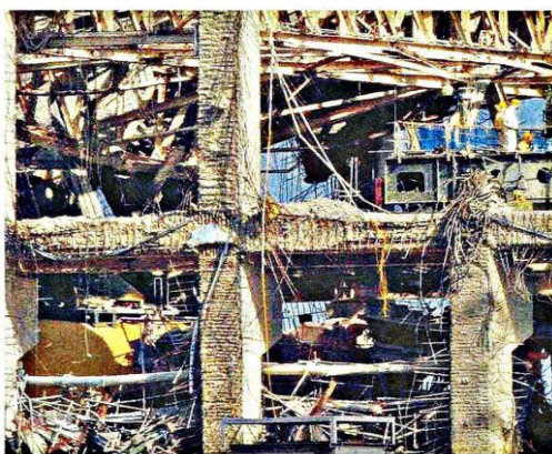
Fukushima Daiichi Reactor #4 after hydrogen explosion
